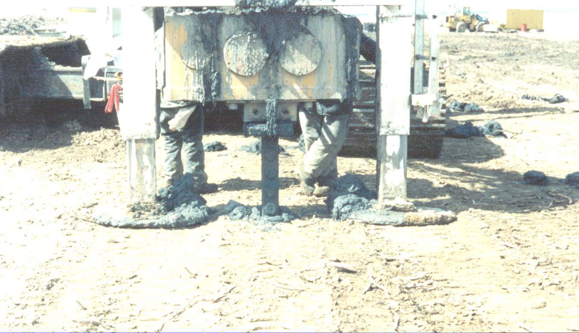
APE bottom drive driving wicks at Craney Island August 2000
