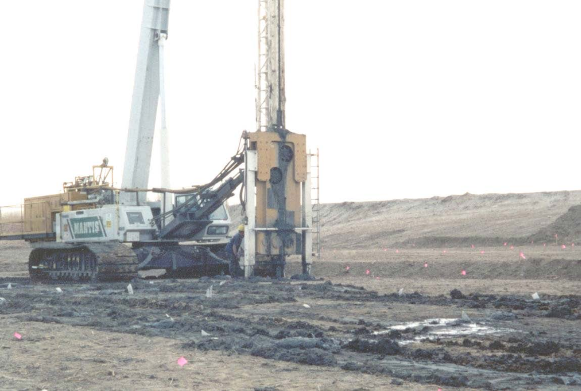
APE bottom drive mounted to Mantis 70 ton crane
