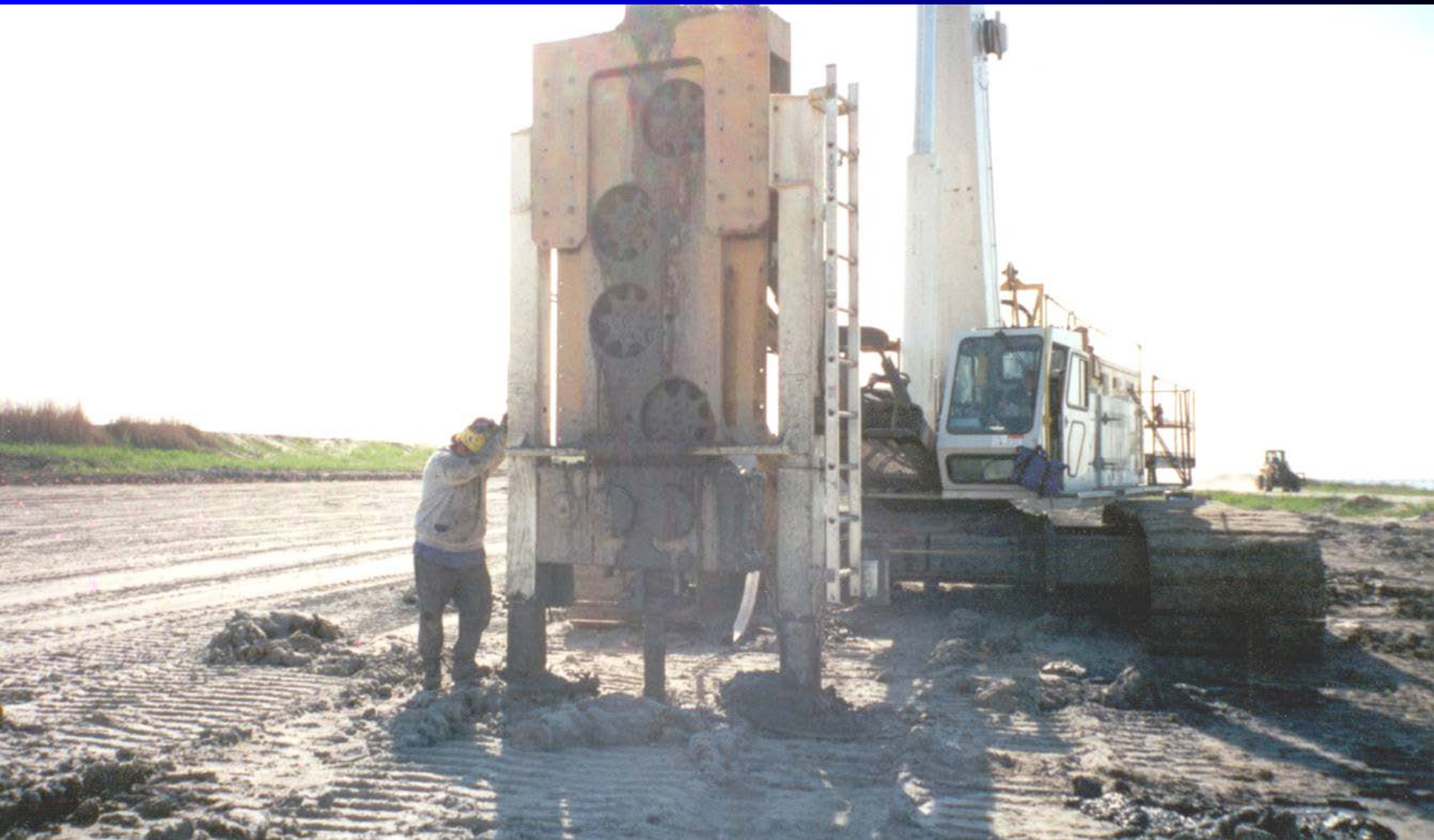
APE bottom drive at Craney Island August 2000
