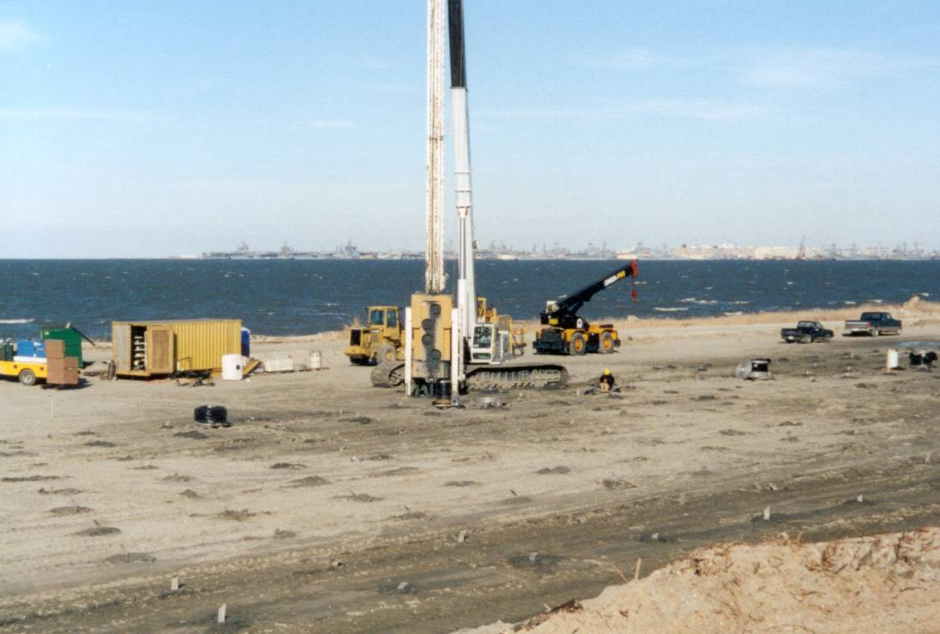
APE bottom drive wick machine working at Craney Island August 2000
