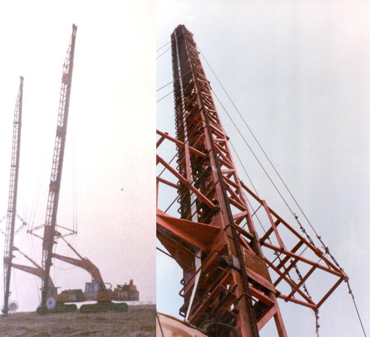
Static rigs working in Hong Kong
