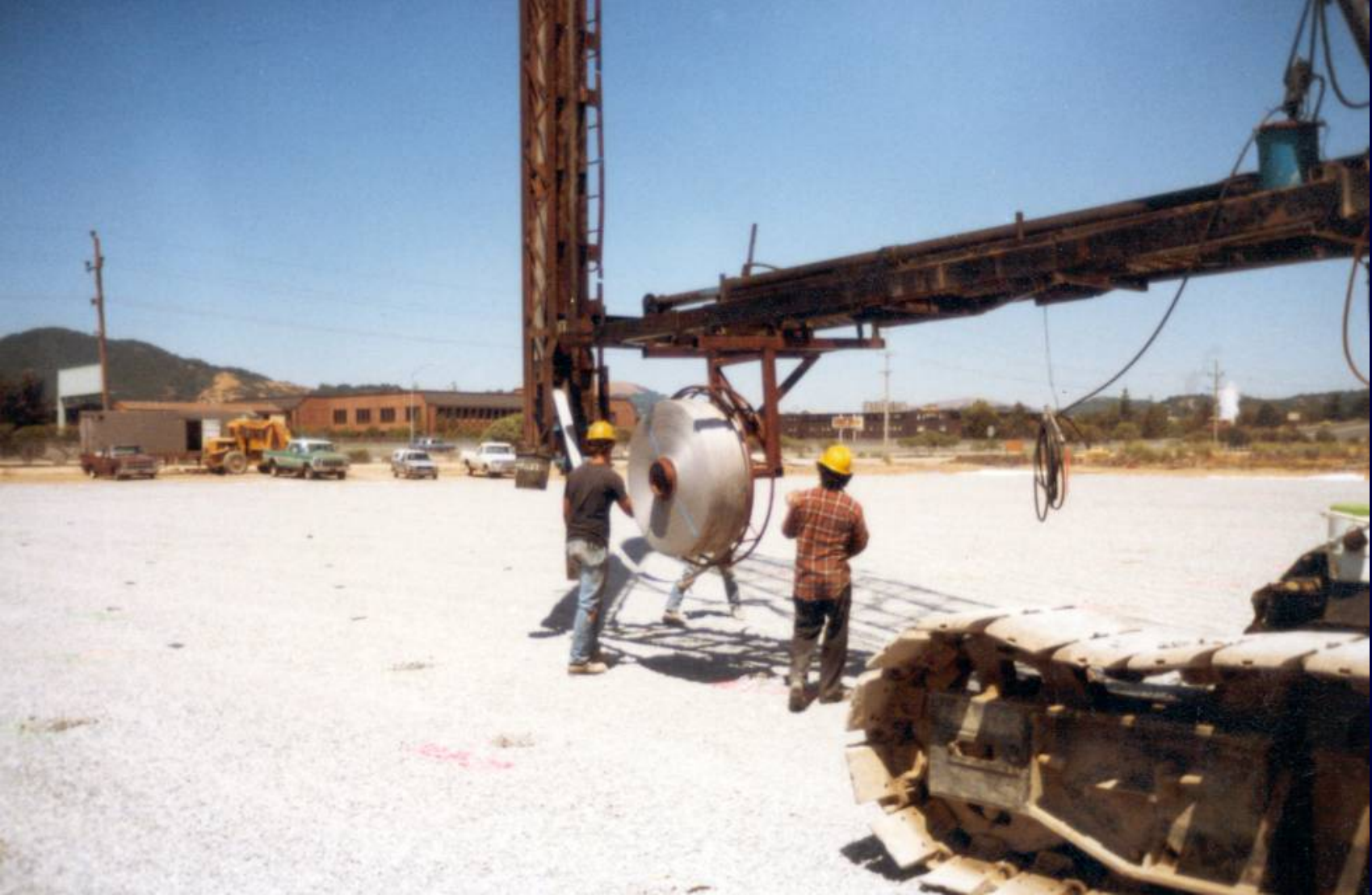
Top Drive vibration only wick installer using crawler crane
