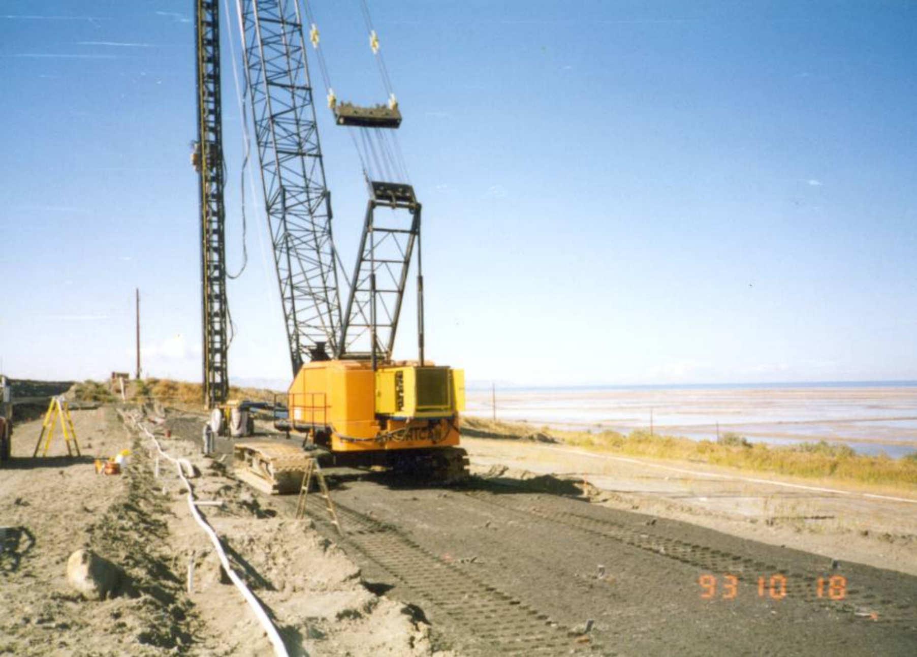
Another view of APE equipment in Salt Lake. Top drive vibro only. Note that APE power unit is mounted on back of 300 ton crane.
